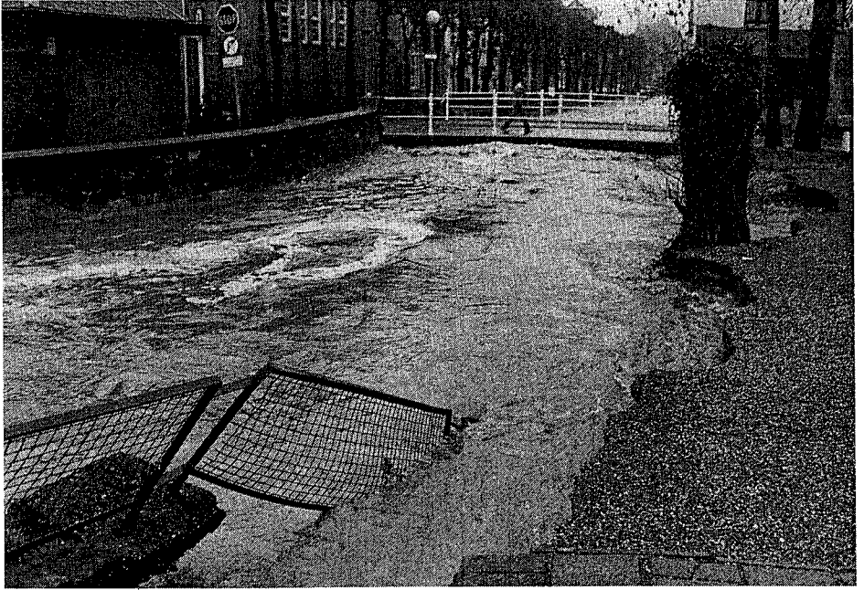
Photo 9.1 Collapsing river banks during a flood in the village of Valkenburg.
